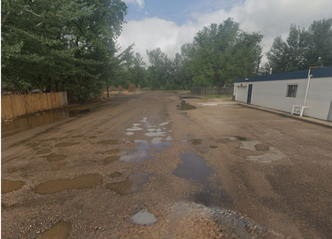
Alpine Street and College Avenue (looking west)
